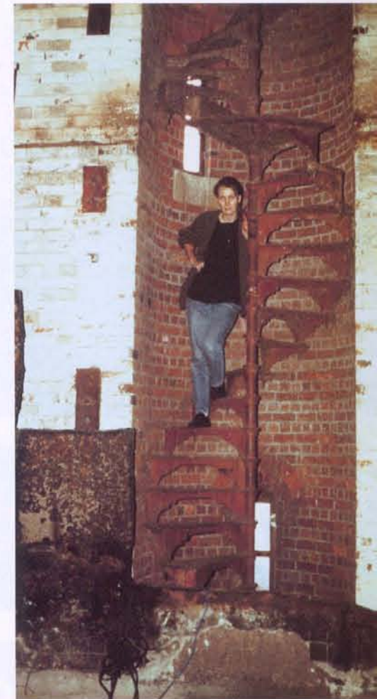
When Godalming-based architect Elspeth Beard bought Munstead Water Tower for £121,000 at auction in October 1998 she became the proud owner of a Grade II listed building that had stood derelict for nearly 20 years and came complete with a 2ft layer of pigeon droppings
